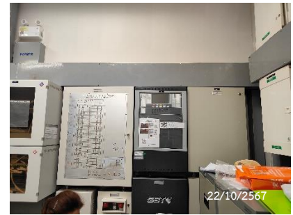
Fire Alarm Control Panel
