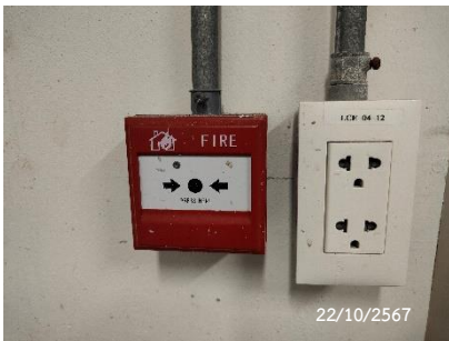
Fire Alarm Manual Call Point
